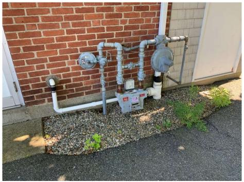
Photograph 8: Natural gas connection and roof drain/sump pump connection to underground reinjection gallery on southwest building corner.
