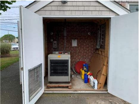
Photograph 5: Natural gas generator within attached unfinished shed.
