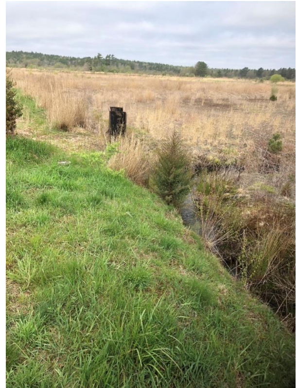
Photo 6: Perimeter ditches direct flow away from bog interior. Note upland grasses within bog cells.
