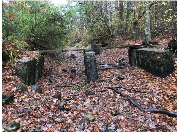
Photo 4: Diversion canal under no-flow conditions 100 feet downstream of diversion structure.
